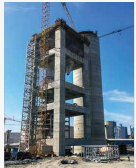
Concrete pumping at 175 m height
