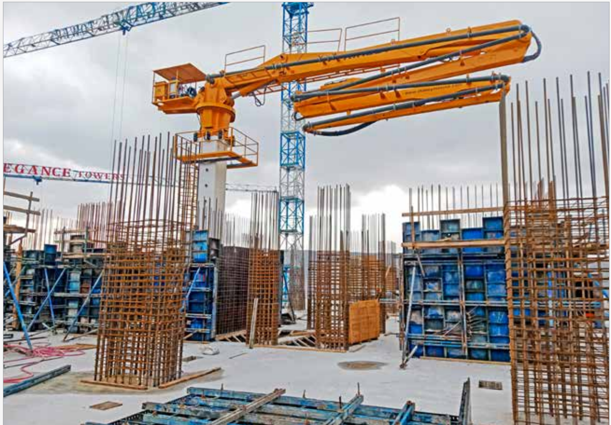
32 Meters 4 Boom Climbing Type Concrete Distributors
