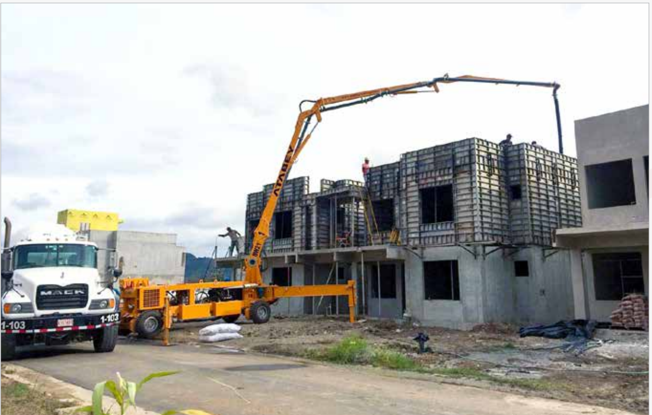
BW Series: 4x4 mobile concrete distributor, closer to perfect mold
