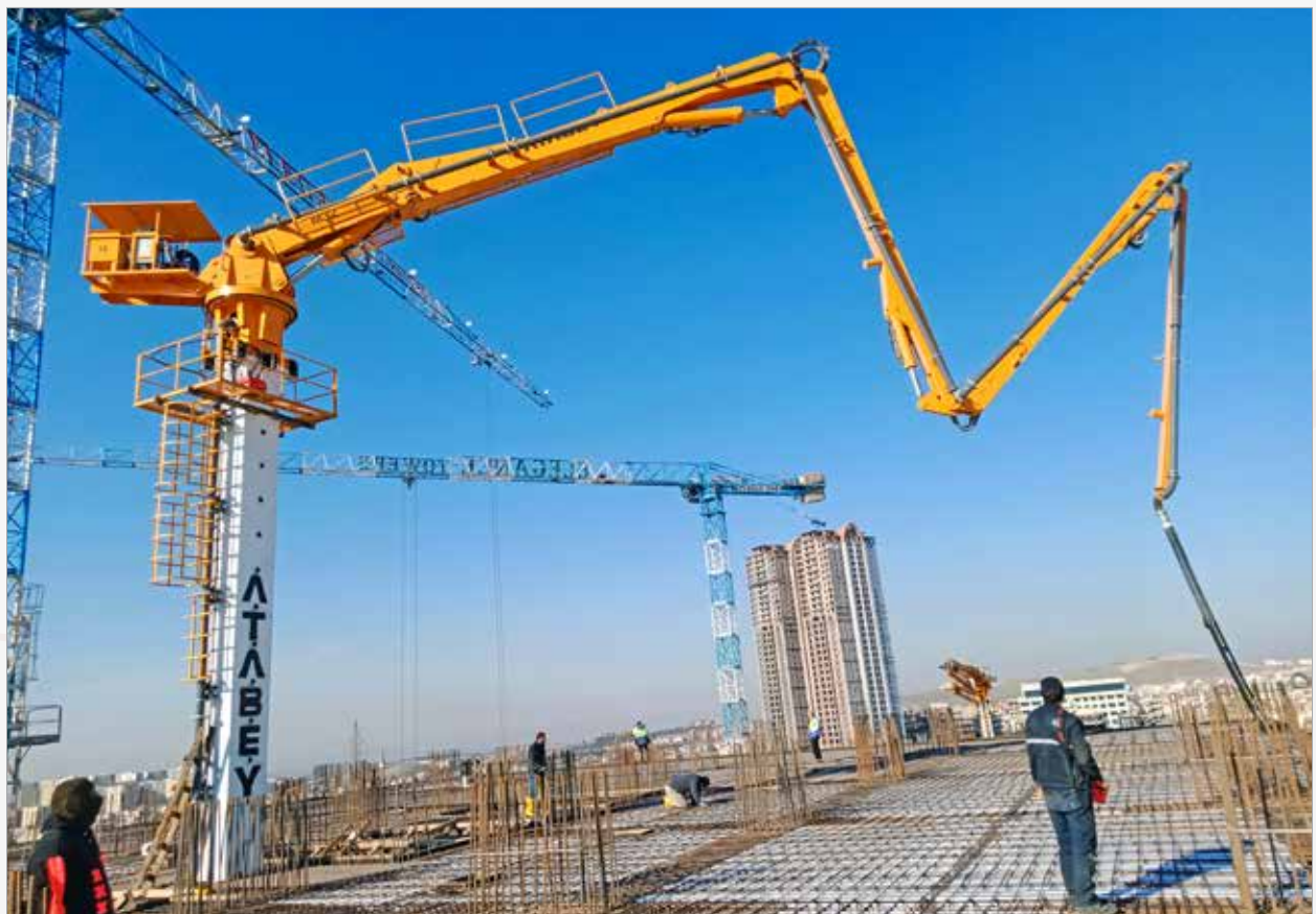
32 Meters 4 Boom Climbing Type Concrete Distributors
